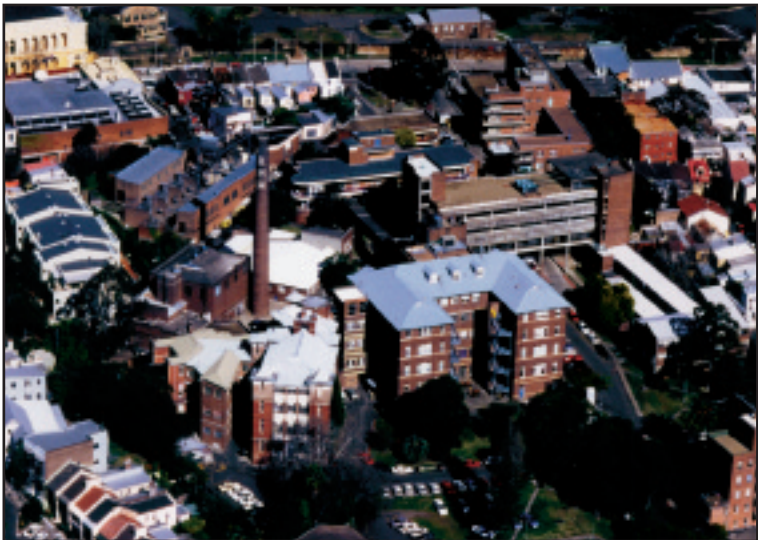
The Royal Hospital for Women shortly before its demolition
